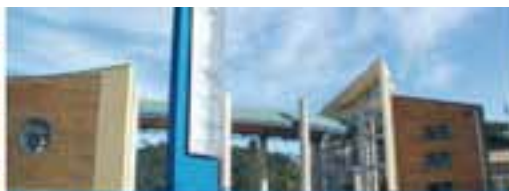
CAMPUS PUERTO MONTT
